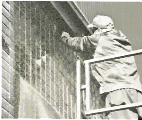
Installation of the cleaned and restored window at 7 South Montana.
