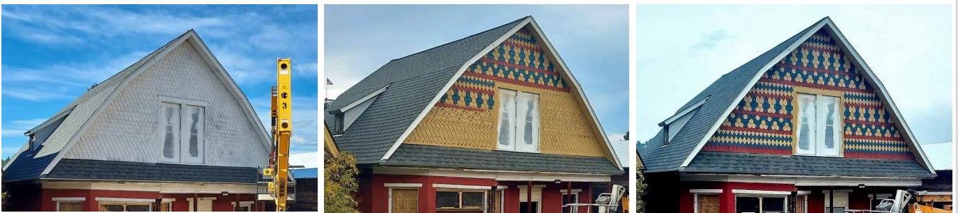
A new paint job on a warm October day brought out the amazing original design of the architectural shingles.
