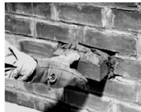
Replacing deteriorated brick
