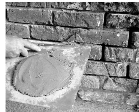
Packing new mortar into joint
