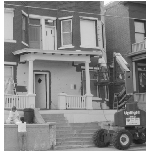
Painting in progress with help from lift.
