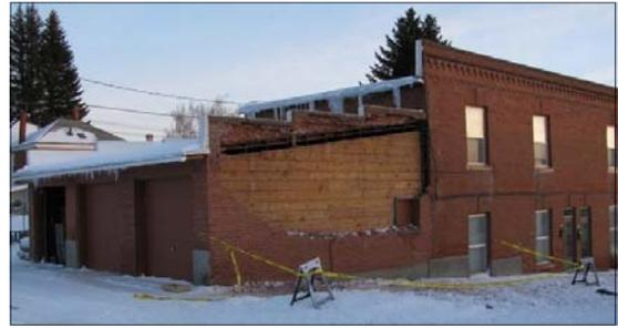
*Catastrophic failure of a historic brick wall during a winter windstorm in Butte. Read the full story at*
