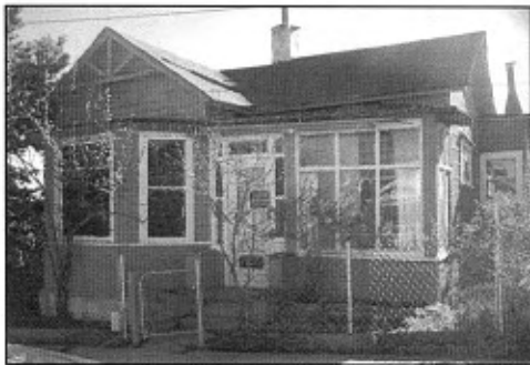
Front view of house. Large front windows designated for glass replacement.
